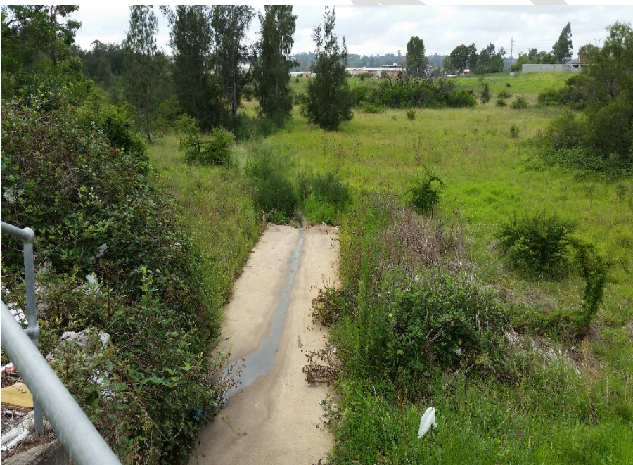
Plate 7 Modified drainage line facing south east
